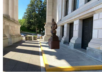
Location 3 South portico Exterior existing slab
